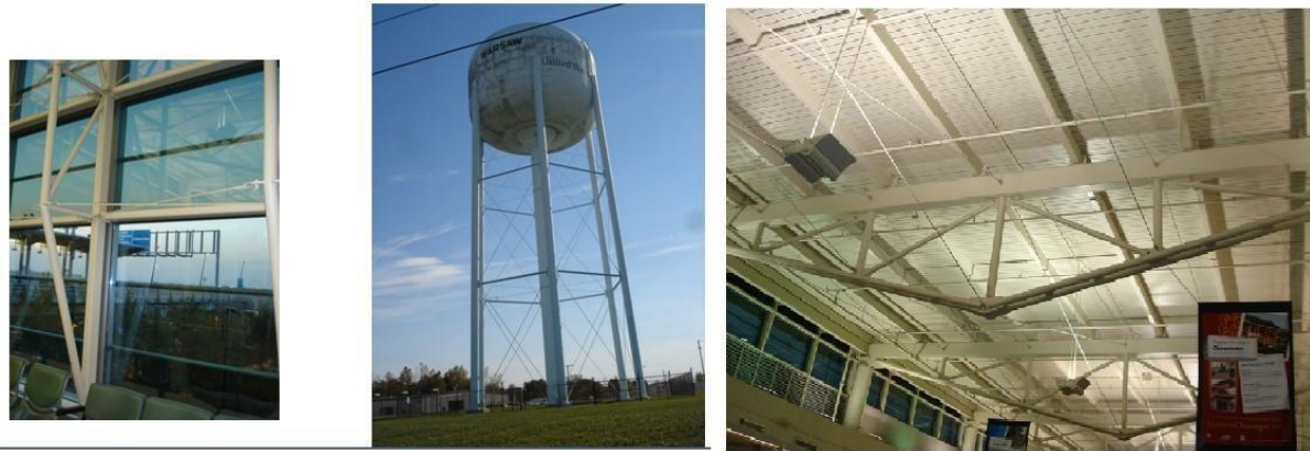
Tie Rods in Structures
